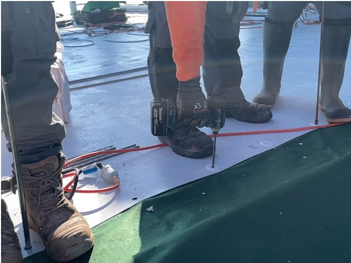
Teamwork makes the dream work! Asphalttec making the installation of the Sika Eject Ecotek telescopic fasteners a breeze.
