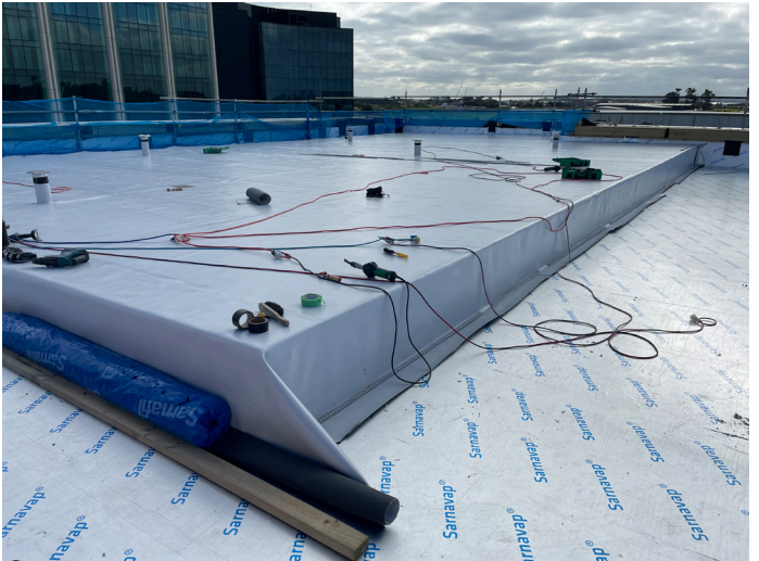
A completed section of the Sika Warm Roof system, awaiting connection to adjacent areas.
