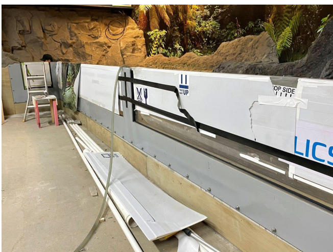
Lobster tank – Viewing glass and frame positioned on nib formed with Sika Monotop-438 R bonded with Sikadur-32. SikaSwell A bonded with SikaSwell S-2 used between nib and concrete base. Sikaflex-11 FC used as a gasket seal between Sika Monotop-438 R nib and steel frame.
