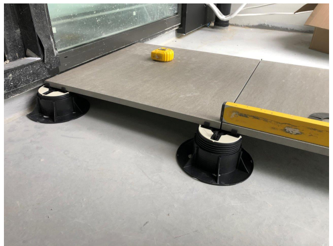
Placing tiles over Sikafloor®400 N Elastic, cured
