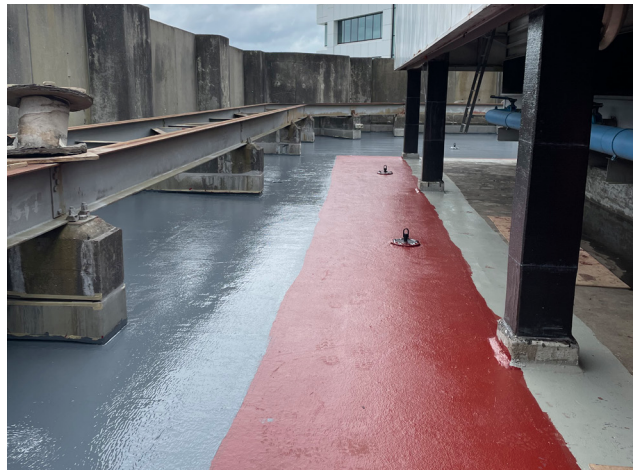
SikaRoof i-Cure Basecoat (Red) has a layer of fibreglas reinforcing imbedded within it. The Topcoat (partially applied) is Slate Grey.
