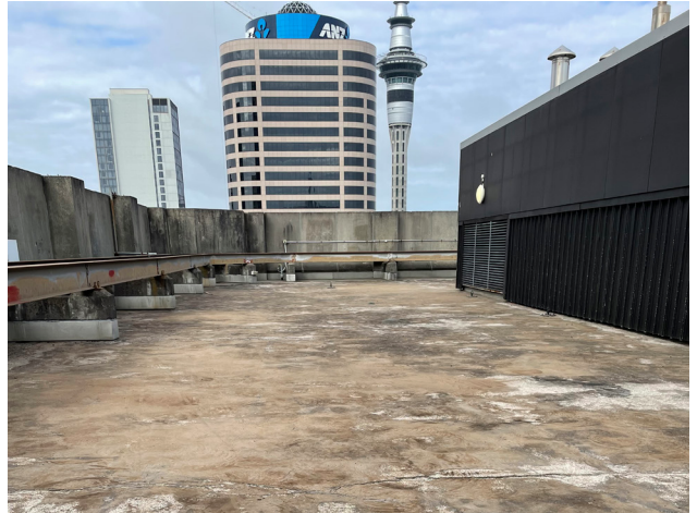
During the preparation of the surface, the original asphalt had to be removed and cracks repaired.
