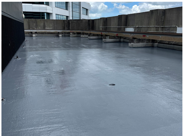
Completed. A seamless, waterproof membrane.
